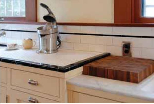
**Kitchen counters** were built in two heights and two materials, the shorter topped in marble ideal for Ann Nitzan's baking, the taller made of hexagonal tile. Backing is flat subway tile, trimmed in black.
